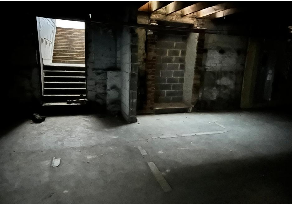
1879 BUILDING / STAIRS OF 1908 BUILDING
