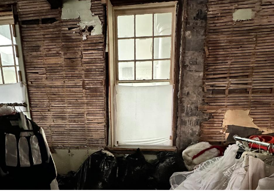
1908 BUILDING - EXTERIOR WALL
