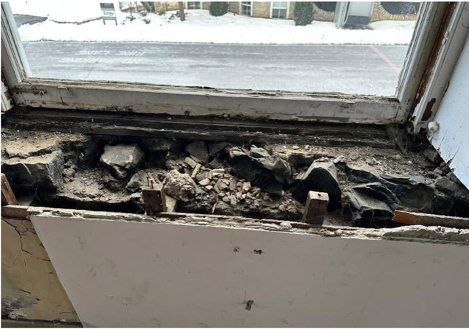
1908 BUILDING - WINDOW SILL
